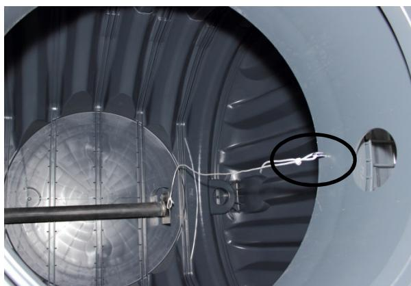
To attach the cord, a hook is fitted inside the tank dome. The hole for the hook should be pre-drilled with a 4mm bit.
