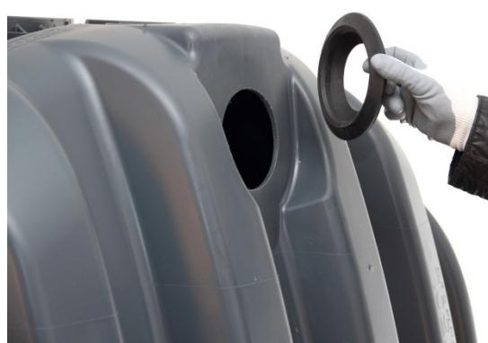
Deburr hole. Insert DN 100 edge seal. The feed-through direction can be seen in the previous diagram.
