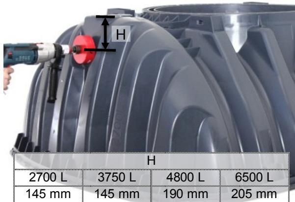
Drill holes for the inlet, outlet and connecting lines on the shells using a DN 100 core drill (diameter 124 mm).
