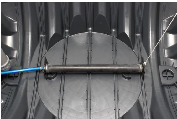
The pipe aerator(s) are positioned on the tank base. To attach the cord, the hook is fastened to the telescopic dome shaft.
