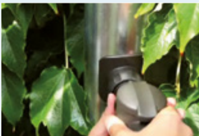
The downpipe is connected using a downpipe filter.
