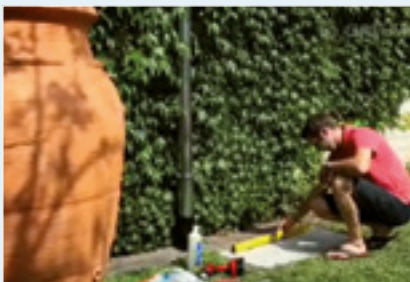
The ground must be level for the installation of a tank.
